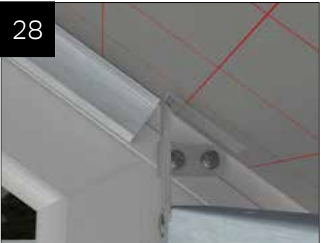
where panel adjacent to the gable is solid - the channel spans from insulated internal pelmet frame up to ridge detail and should be fitted directly below the 90mm insulation (insulated internal pelmet detail shown).
