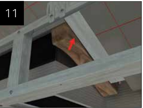
In the case of an L-shaped conservatory, where the box gutter returns around the house wall If the distance between the side gutter fascia and the adjacent transom bar is less than 100mm, 90mm insulation will not be specified and a gap will remain- in this case, insert mineral wool to fill the cavity.
