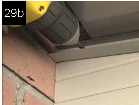
Mono pitch detail shown - channel terminates at host wall.
