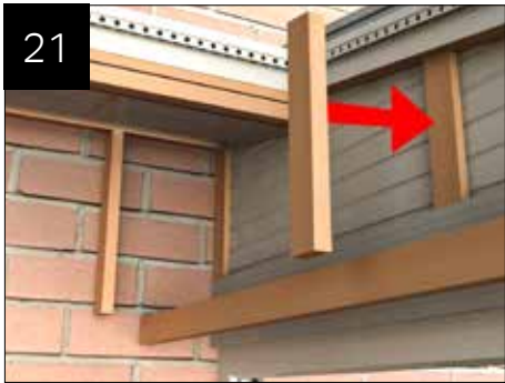
Add a framework of 25mm x 44mm battens this should consist of 1 horizontal batten along the lower edge of the eaves fascia and uprights stacked on top of the 13mm verticals installed in step 15.
