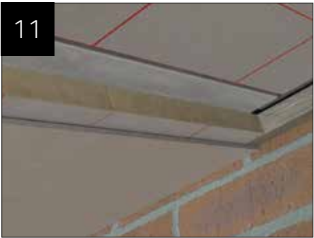
When fitted, the 25mm insulation should butt up to the batten, and the plasterboard should fix through into the underside of the batten as shown.
