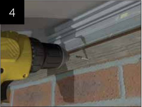
It may be useful to fit an angled batten at the host wall - this will provide a positive fixing point when fitting the plasterboard.
