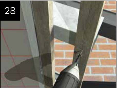
Fit second row of battens as described on page 40.
