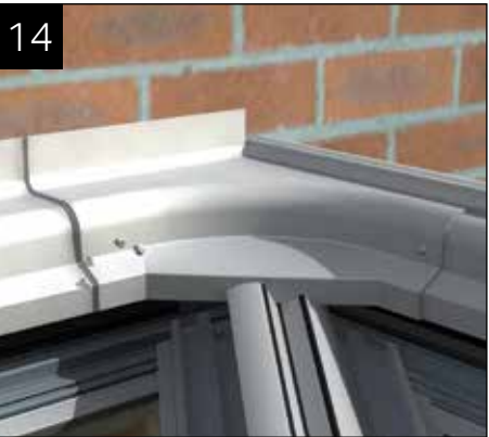
The joint between the full and half ridge PVCu top caps is sealed by the use of a capping connector. This needs to be trimmed to suit. Bed the capping on suitable sealant and fix using the plastic rivets provided.
