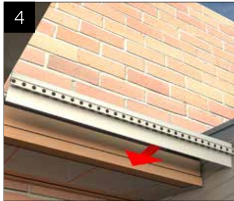
Fit LVCT600W and ensure it touches glass. Screw fit using drywall screws) along the lower edge.
