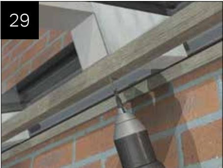
Fit additional battens where glazing is present along the host wall as shown.
