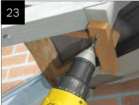
Fix into position using plasterboard screws. NOTE: when fitted, the battens should terminate at the centreline of the steel undercladding to allow for fitting of the adjacent panels
