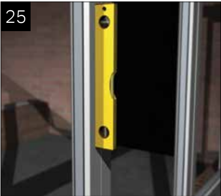
Ensure the window frames are plumb.
