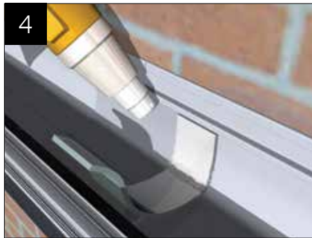
Check surfaces are dry, clean and grease free. De-grease if necessary. Heat both the sealing tape and the box gutter with a heat gun and position the tape over the joint. Press the tape firmly across the joint of the sleeve and the box gutter ensuring there are no air pockets.
