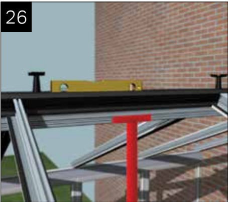
Ensure the ridge is level.
