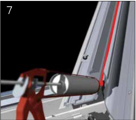
Now run a continuous bead of suitable sealant down the entire length of the aluminium valley profile, at the point of the hinged connector in the centre.
