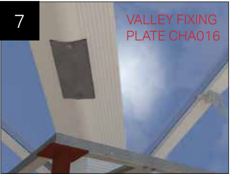
Mark out and cut the valley cladding and fix valley fixing plate by following steps 1 - 5.
