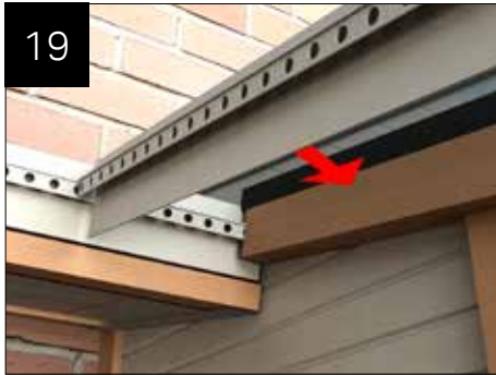
Fit LVCT600 trim, covering timbers and enclosing LFS600 black plastic trim- again, ensure it touches the glass and fix using drywall screws.
