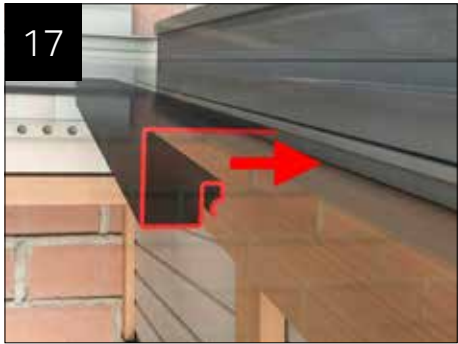
Slide LFS600 black plastic trim into place between the glass and timber battens as shown. This creates a solid black detail when viewed from the outside.
