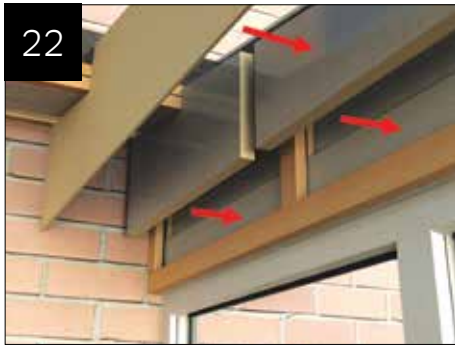
Fill the cavities between the timbers with 25mm insulation and finish with plasterboard.
