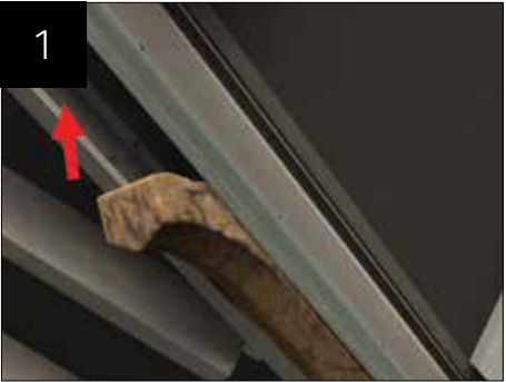
Insert mineral wool (LVIR001) between the valley wings along the whole length to insulate the cavity.
