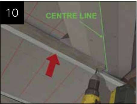
Fit the ridge battens, as described on page 39. NOTE: On the valley side, the batten should terminate on the valley Plate centreline as shown.
