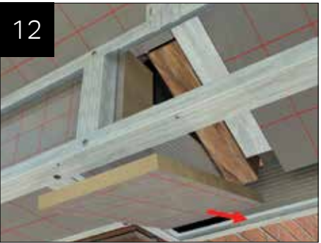
Fit 25mm insulation adjacent/beneath gutter around the return as shown in step (10) to help prevent cold bridging. Remember to fully insulate the entire internal pelmet with mineral wool supplied.
