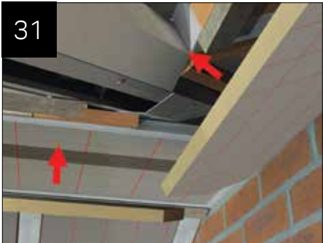
Fit 25mm insulation.
