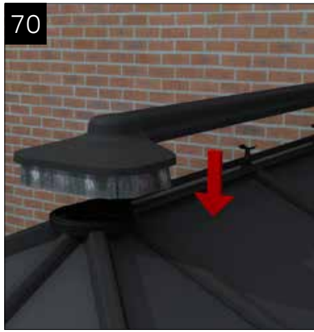
Offer up the complete ridge capping onto the roof.
