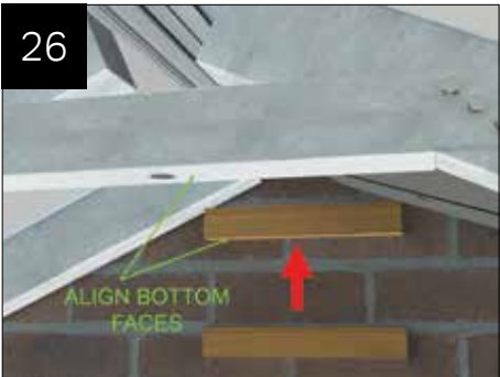
Fit a length of timber batten to the host wall, ensuring that its underside lines through with the underside of the struts (LVTS001/LVTS002). This will provide a fixing point for the ridge board fitted in the next step.
