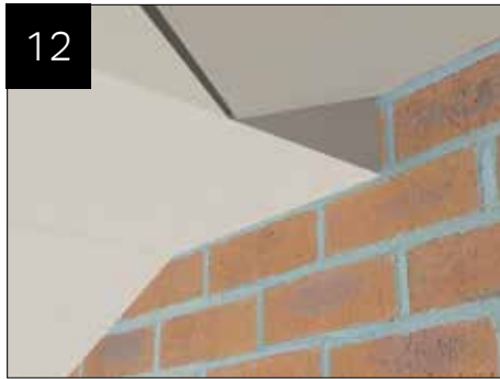
Now fit the plasterboard – the detail where the valley abuts the host wall should look as shown.
