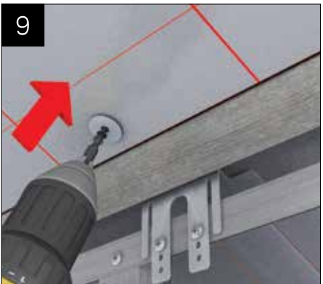
Fasten through the board and into the glazing bars using the drywall screw provided (3.5 x 50mm) and with a washer (kit of 25) behind the head to offer additional support to the board. Use location plan to identify board positions. Use tape LVFT045 - foil sealing tape - tape ALL joints of 25mm insulation.
