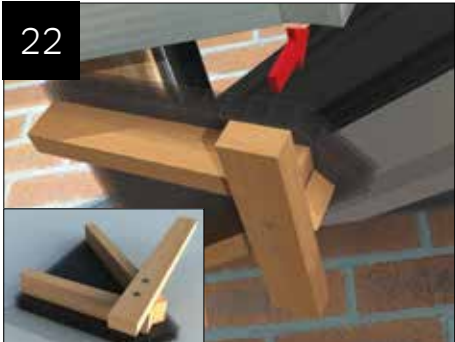
Offer up the cassette assembly into position.
